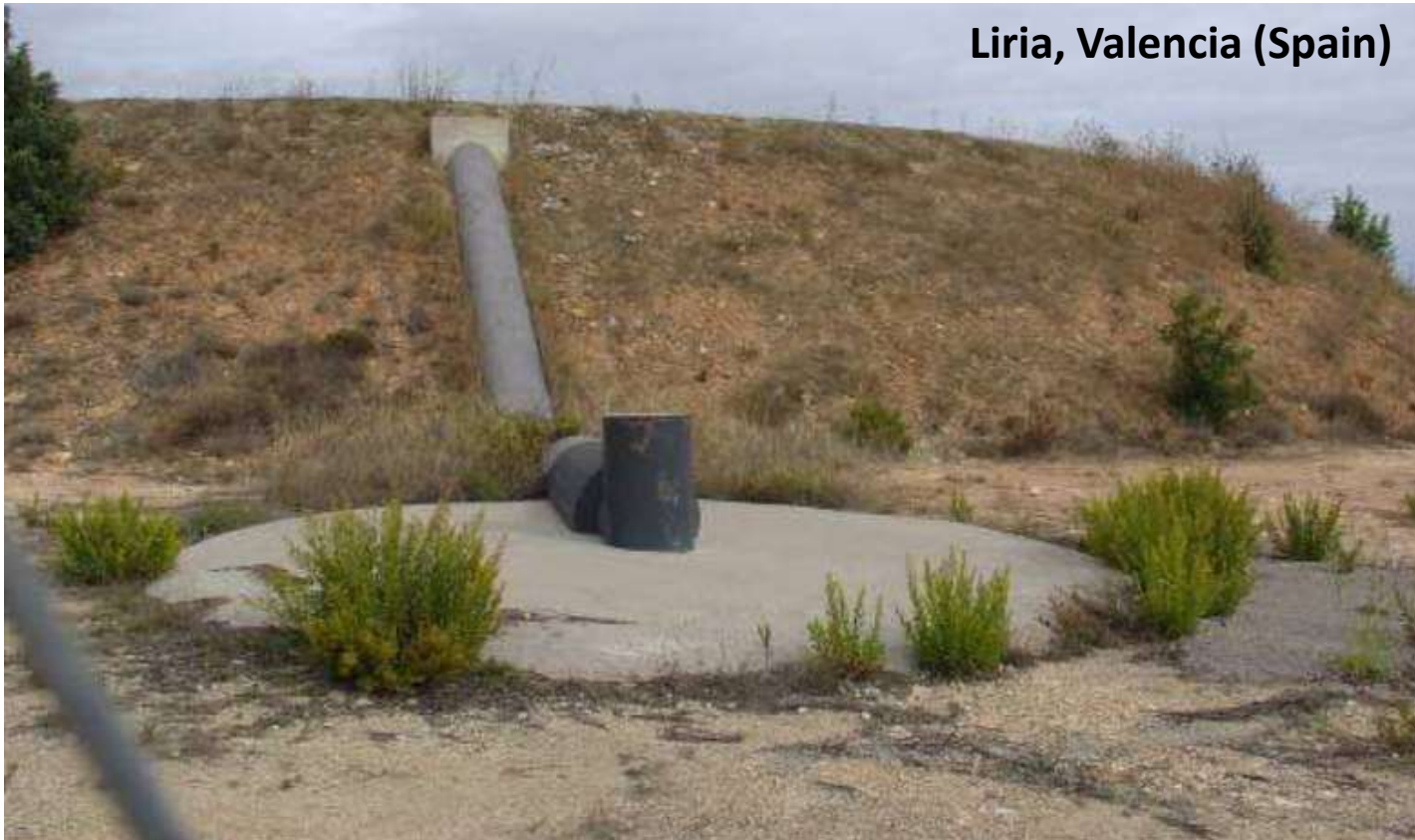
MAR borehole associated to an Irrigation pond
